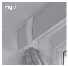
Fit the cassette back into the recess ensuring it is a snug fit and fold the lever bracket down to secure the blind (Fig.  $6\ \&\ 7$ ).
